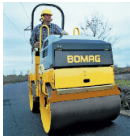
BW90AD-2 in action on an asphalt repair
